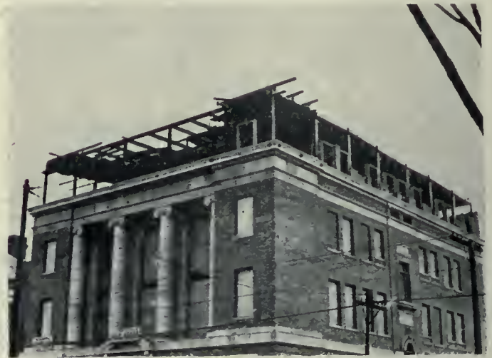
Fig. 4.—Administration Building, Toronto. Erection Progress Jan. 6.
